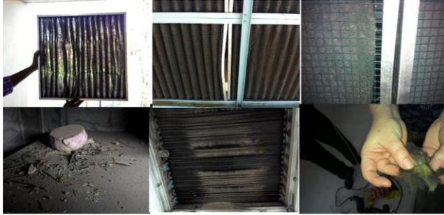
Fig. 3 There were lots of problems with current ventilation system operation and filtration.
